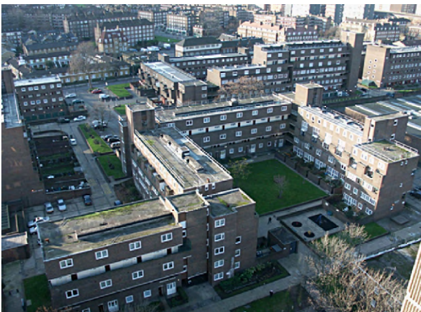
Fig. 7. Original flat roofs at Ethelred Estate and green sedum roofs after refurbishment.
