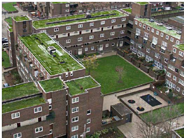
Fig. 7. Original flat roofs at Ethelred Estate and green sedum roofs after refurbishment.
