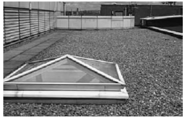
Fig. 8. Rooftop with protective chippings.
