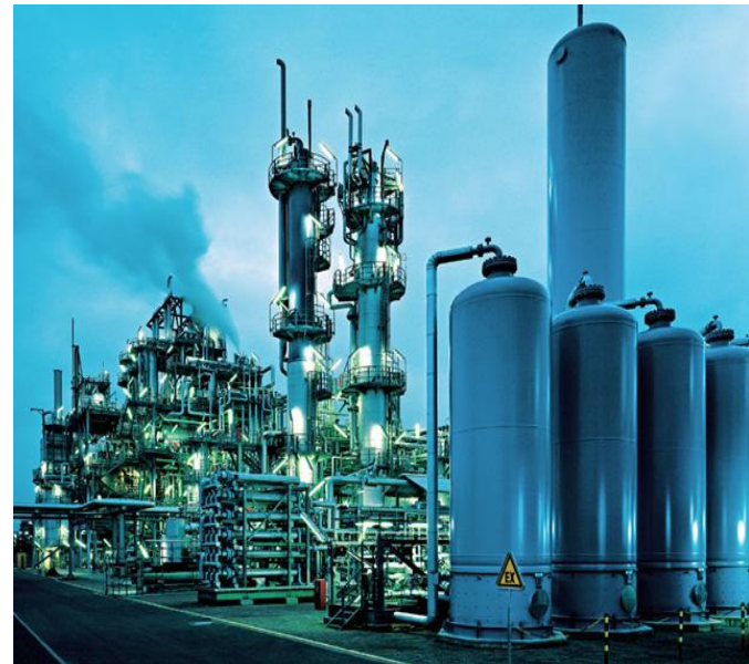
Figure 1. Syngas Plant in Germany. Source http://www.linde-engineering.com/process_plants/hydrogen_syngas_plants/gas_products/syngas.php
