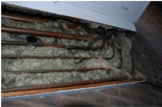
**Figure 6: poor pipe insulation**
