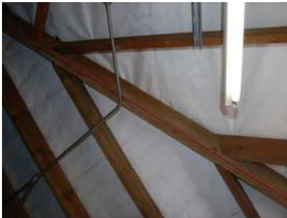
**Figure 8: No roof insulation**
