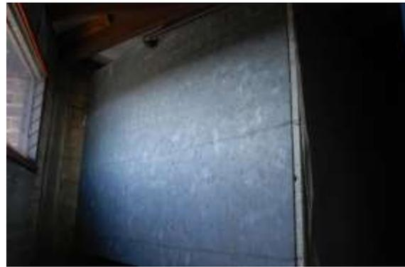
**Figure 7: Water tank with no insulation**
