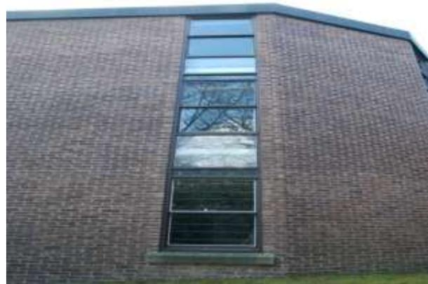
**Figure 3: Large single-glazed windows interior view and exterior view**
